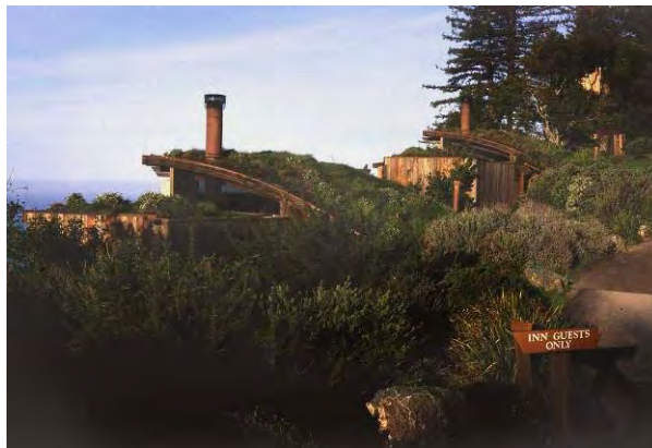
Figure 3-34: Extensive green roof at Post Ranch Inn, Big Sur, CA.
